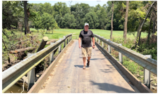
Tim Carlson walks across #11-#13 bridge last week.
